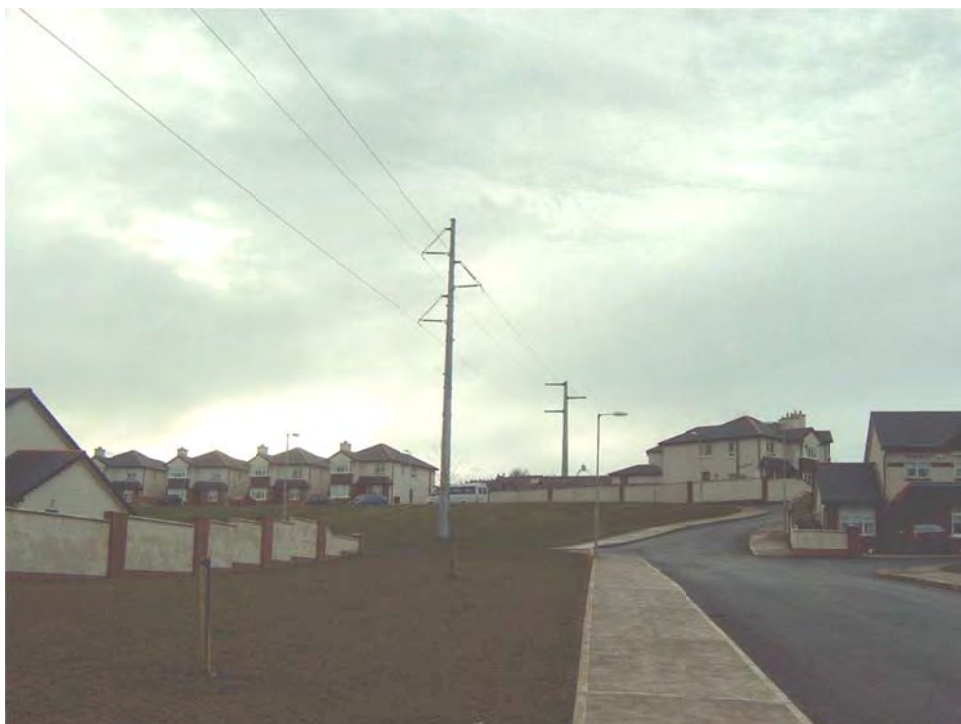
Photo 2: 110 kV Monopole Overhead Line in Cork
